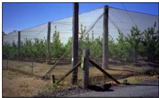
Funding is for full exclusion netting with canopy and sides, to avoid wildlife injuries.
